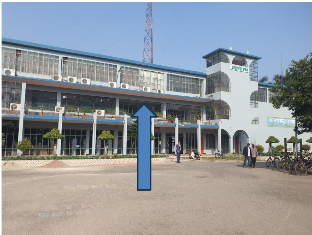
Figure 2.2: Central Library building (UIH will be established on 1st floor)
